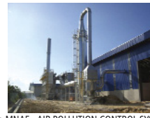
• MNA5 - AIR POLLUTION CONTROL SYSTEM FOR LEAD SMELTING PLANT
